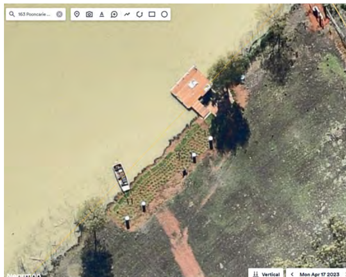
Figure 3. Image of 163 Pooncarie Road Lot 4 DP 1239541 Wentworth dated 17 April 2023. Pontoon (water recreation structure) already constructed.
