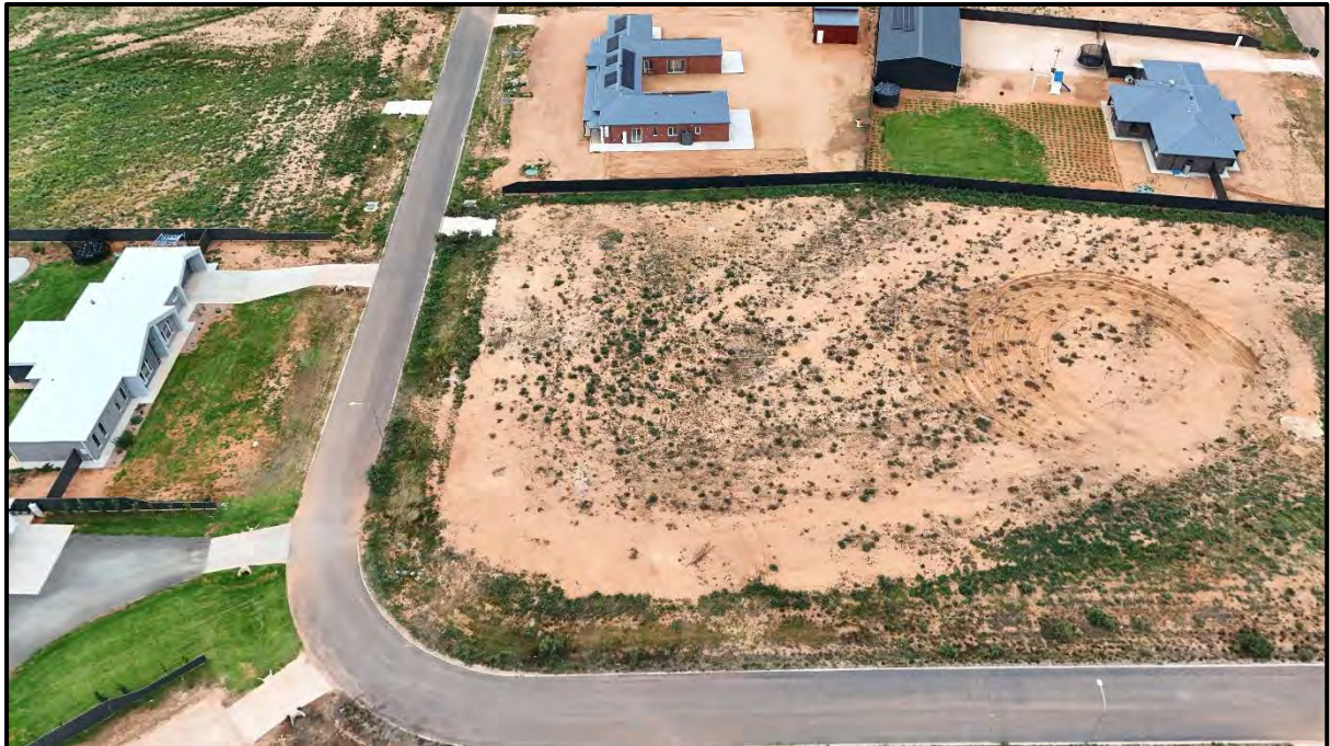
Figure 2: View of site from Wurlong Drive
