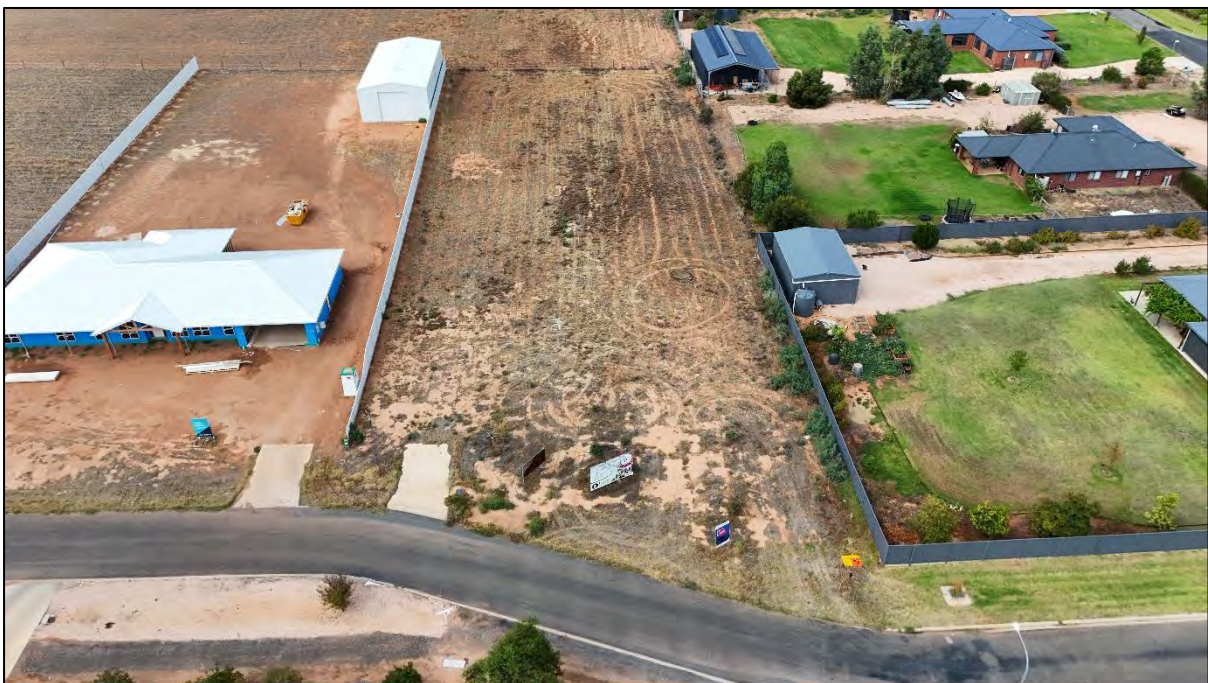
Figure 2: View of site from Wurlong Drive
