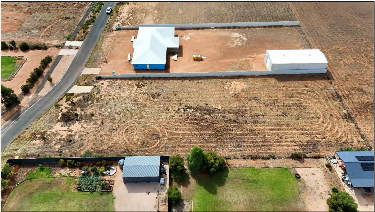
Figure 4: View of the site from the west
