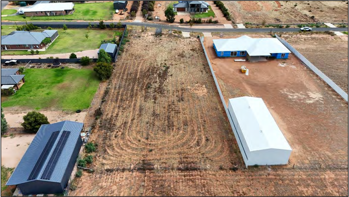
Figure 3: View of the rear of the site
