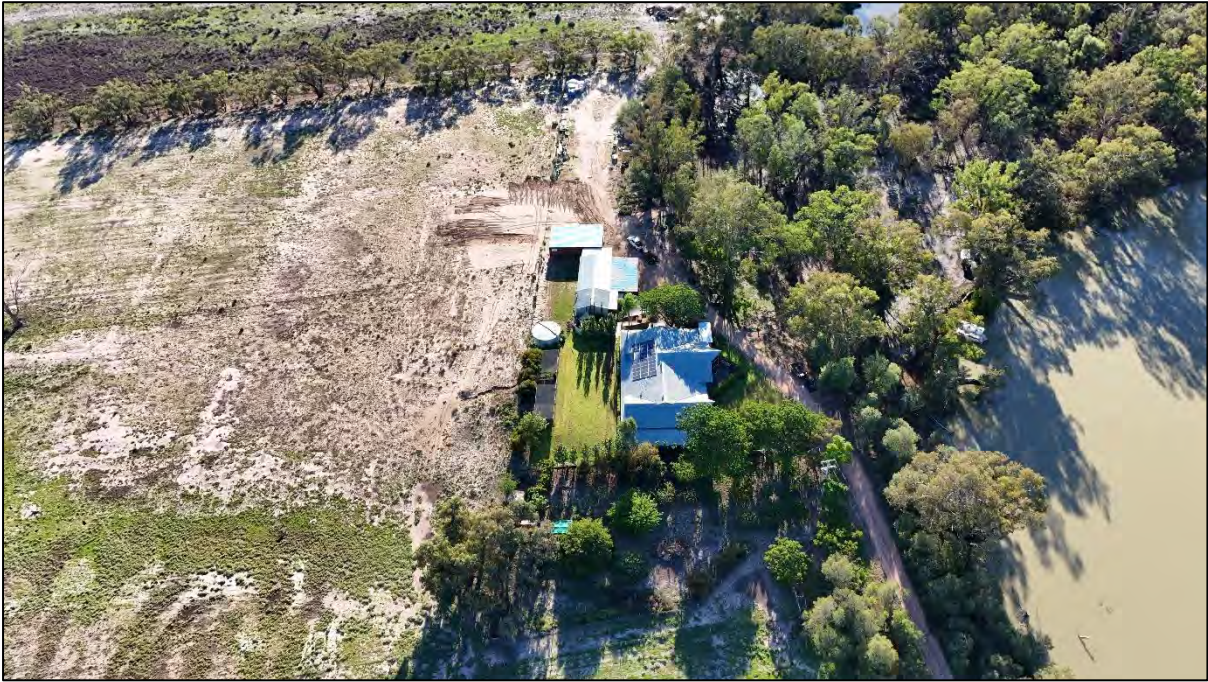
Figure 5: Part view of site from the west
