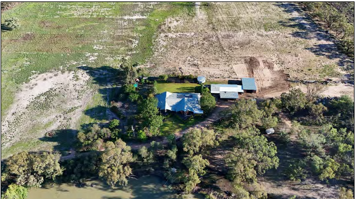
Figure 2: Part view of site from the south
