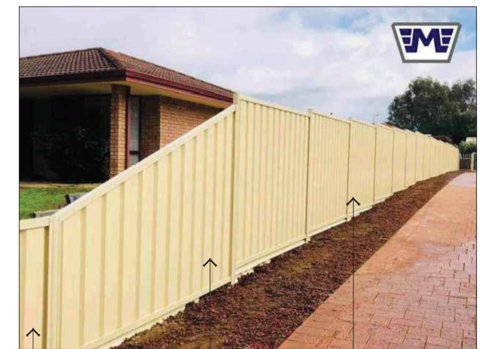
2400mm LONG x 900mm HIGH COLORBOND FENCE PANEL COMMENCING FROM FRONT BOUNDARY LINE. 2400mm LONG TAPERING COLORBOND FENCE PANEL (900-1800mm HIGH) 1800mm HIGH COLORBOND FENCE
