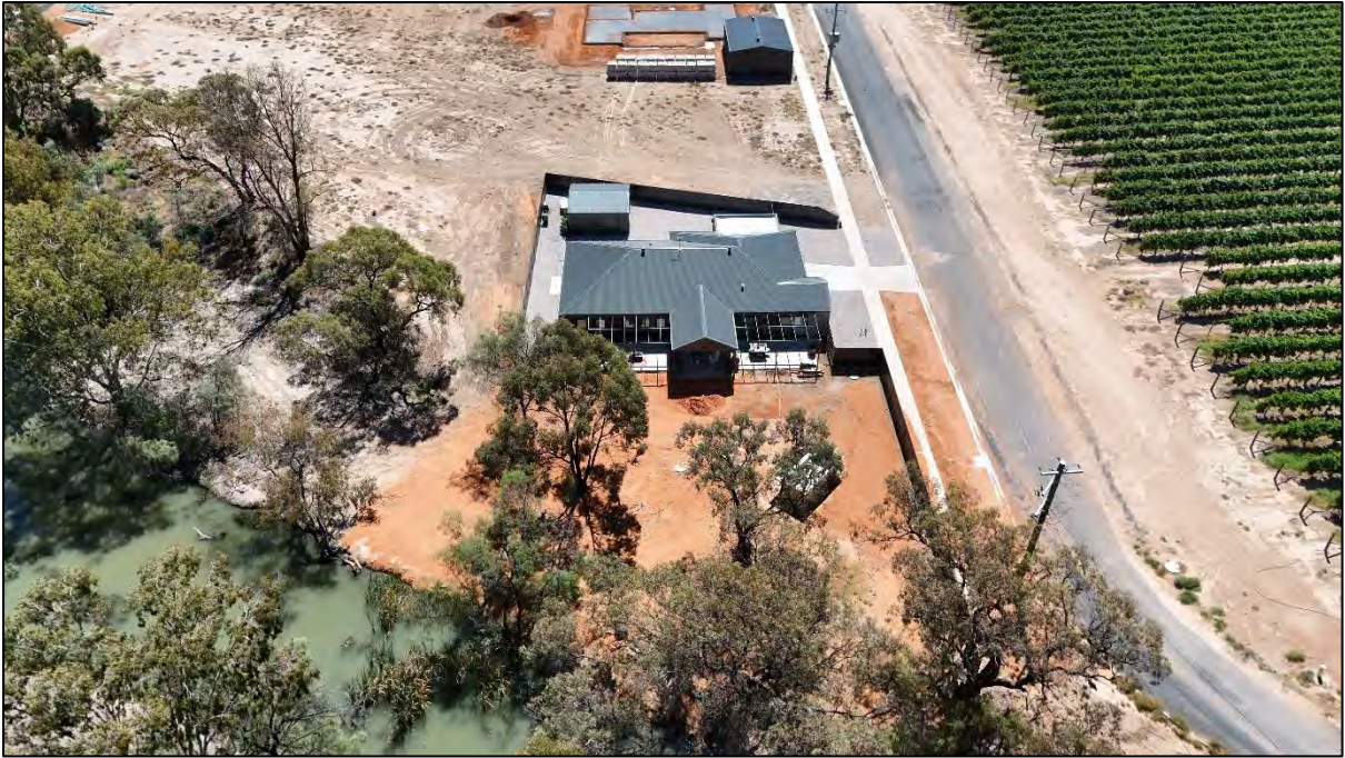
Figure 5: View of the site from the east
