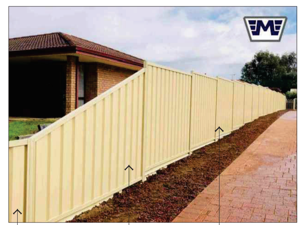
FENCE DETAIL N.T.S 2400mm LONG x 900mm HIGH COLORBOND FENCE PANEL COMMENCING FROM FRONT BOUNDARY LINE. 2400mm LONG TAPERING COLORBOND FENCE PANEL (900-1800mm HIGH) 1800mm HIGH COLORBOND FENCE
