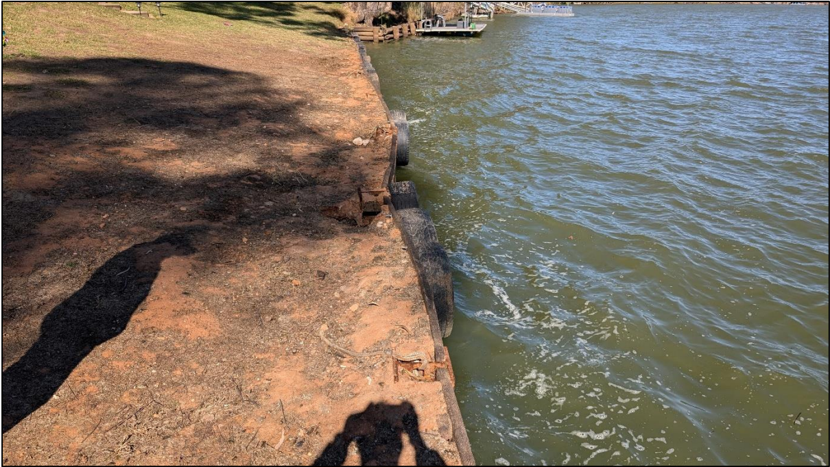
Figure 3: View of the existing retaining wall from the north west
