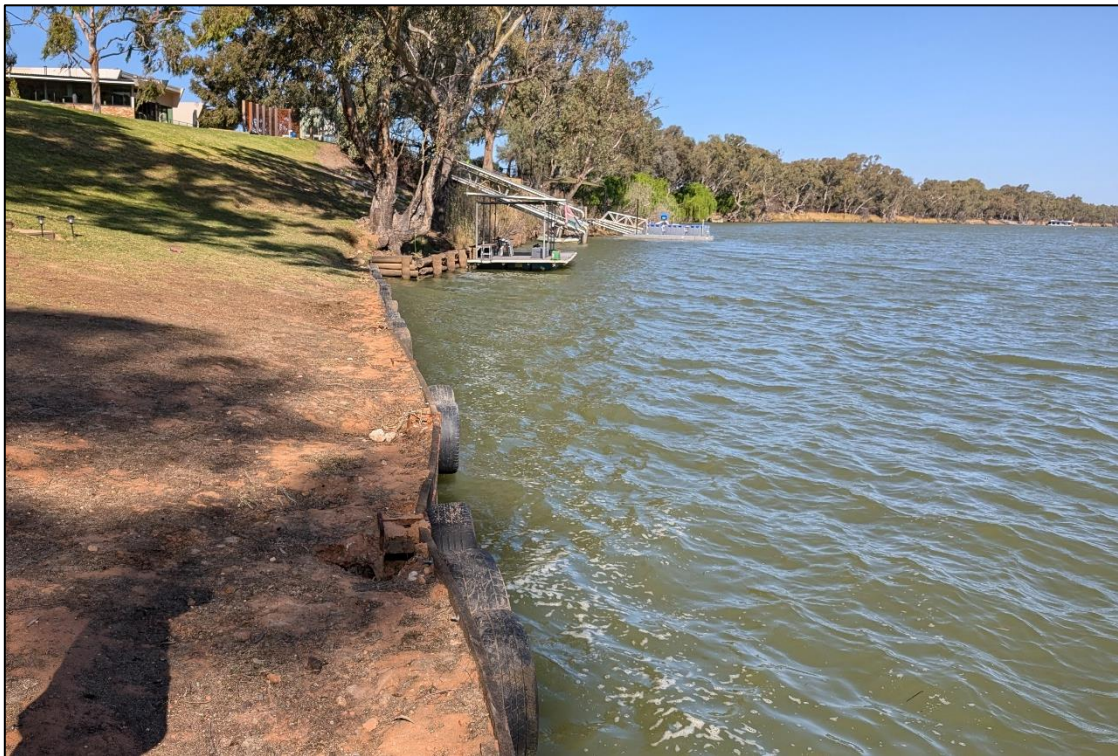
Figure 2: View of the existing retaining wall from the north west
