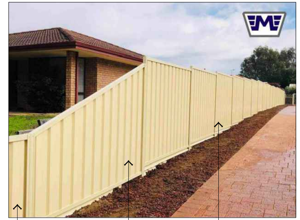
2400mm LONG x 900mm HIGH COLORBOND FENCE PANEL COMMENCING FROM FRONT BOUNDARY LINE. 2400mm LONG TAPERING COLORBOND FENCE PANEL (900-1800mm HIGH) 1800mm HIGH COLORBOND FENCE
