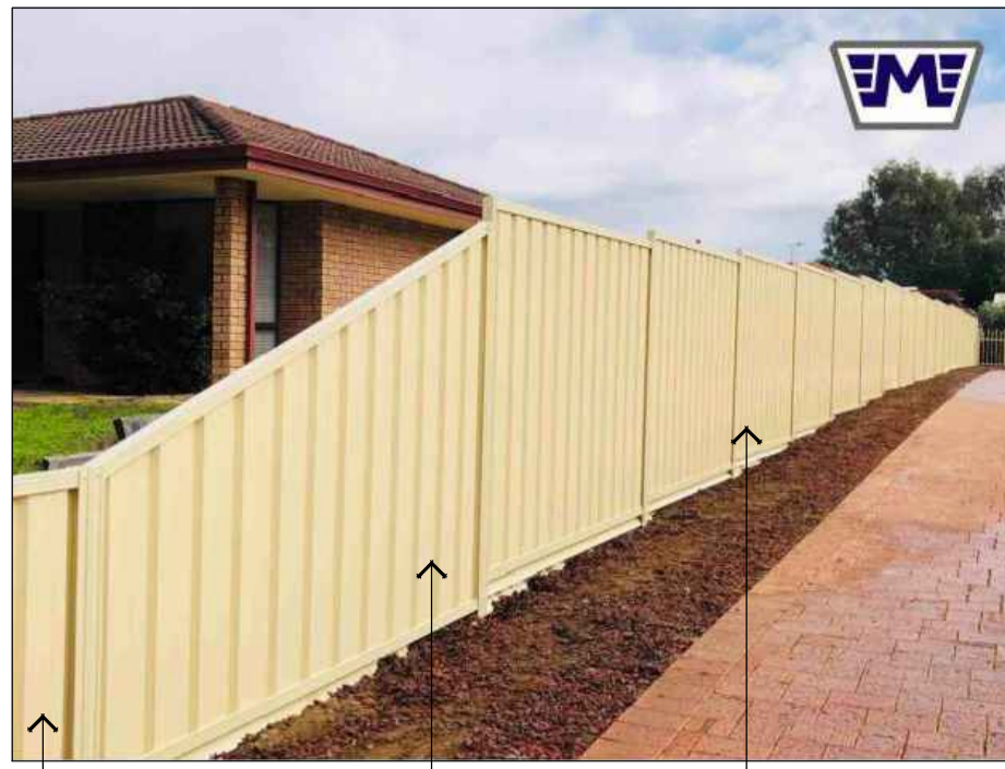
2400mm LONG x 900mm HIGH COLORBOND FENCE PANEL COMMENCING FROM FRONT BOUNDARY LINE. 2400mm LONG TAPERING COLORBOND FENCE PANEL (900-1800mm HIGH) 1800mm HIGH COLORBOND FENCE
