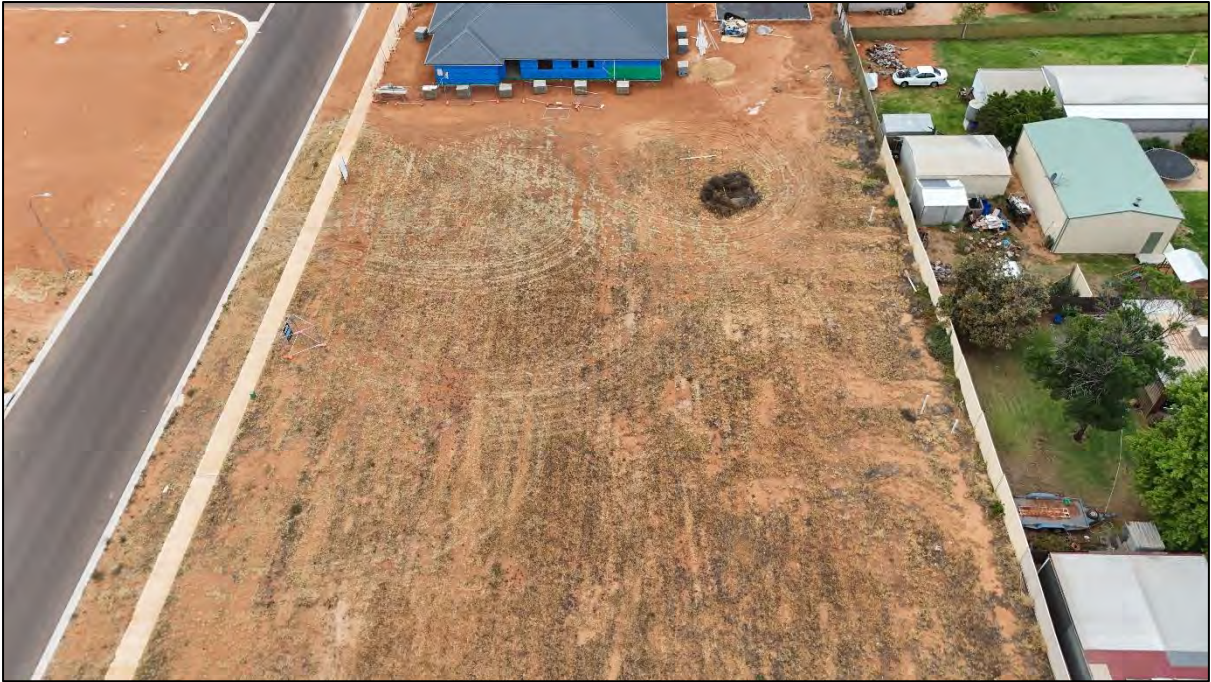
Figure 3: View of the site from the west
