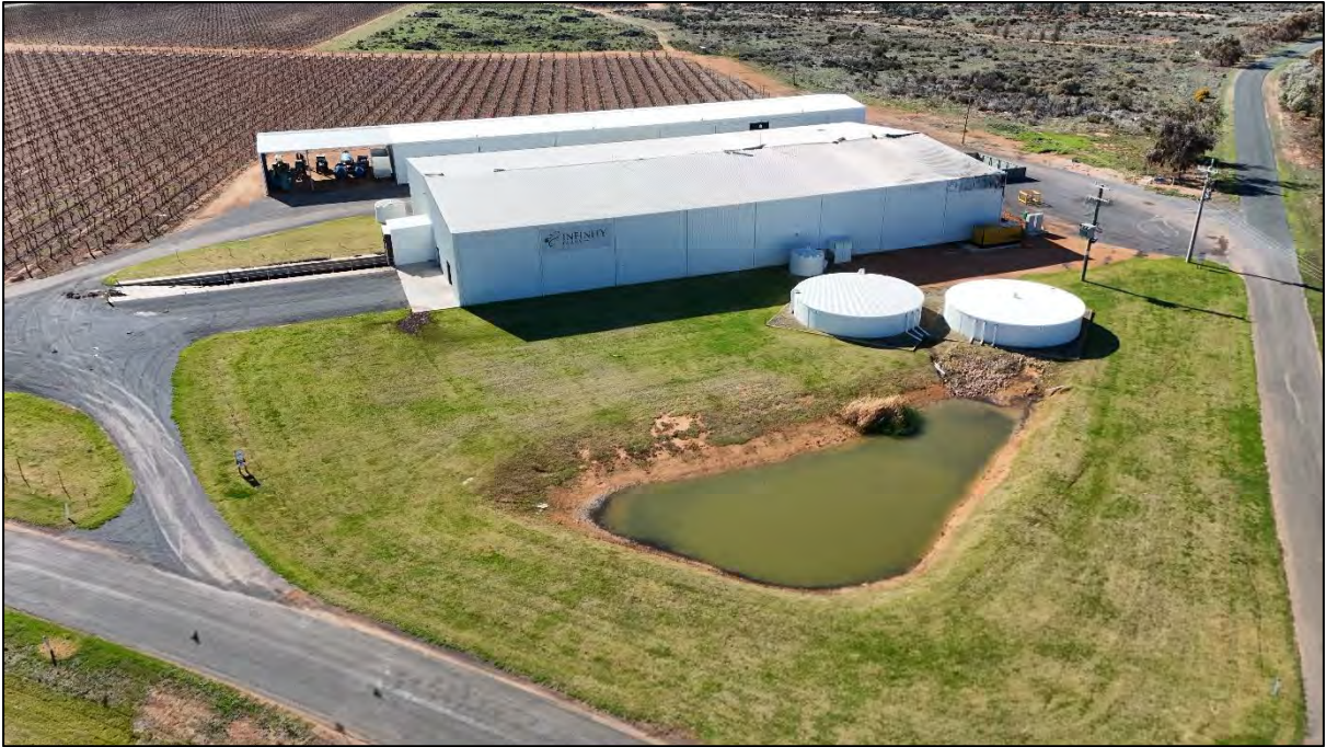
Figure 3: Part view of the site from the west
