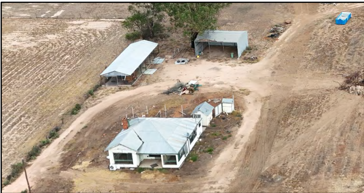
Figure 4: Buildings to be demolished
