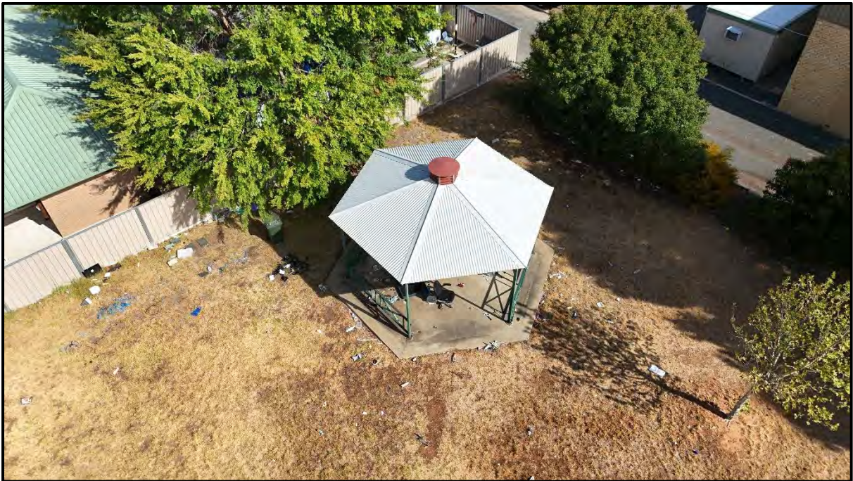
Figure 3: Photo showing buildings to be demolished
