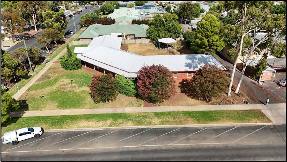
Figure 2: Photo showing buildings to be demolished
