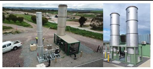
The LMS Gas Flare provides Australia's most proven flare for the clean combustion of landfill biogas. LMS have engineered this technology by drawing on more than 35 years of biogas combustion experience. LMS flares have been purpose built for the landfill environment and their performance in terms of total carbon abated from Australian landfills is unmatched.
