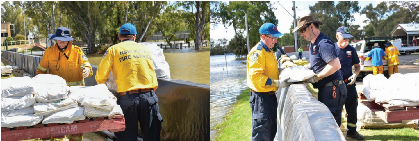
NSW Rural Fire Service placing sandbags at the temporary wall at Wentworth Wharf
