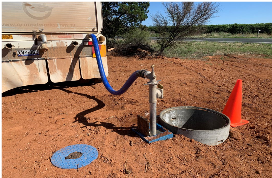
Water truck flushing & disinfecting the main, Mourquong Water Main Extension.
