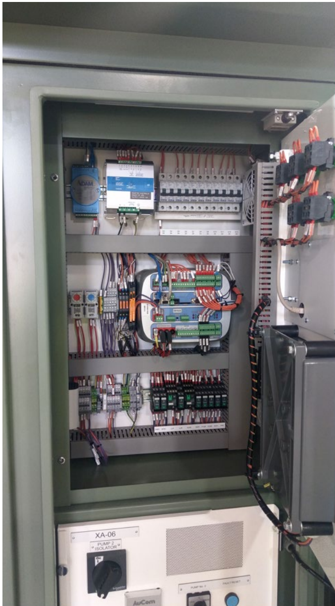
Wentworth Sewer Rationalisation - installation of switchboard and start of telemetry antenna cage installation.
