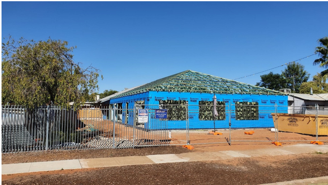
Framing completed and plumbing roughed in
