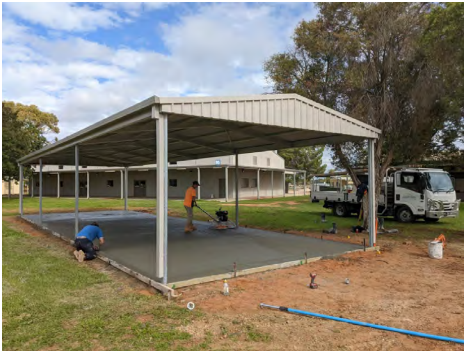
Slab works for the shade structure at the Wentworth Showgrounds
