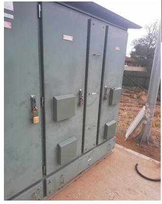
Cooling vents escutcheon with vent holes and outside vent covers- SPS2 (4/02/22)
