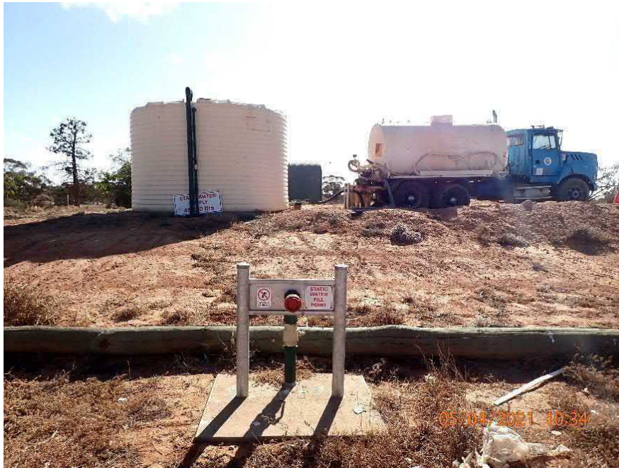
Photograph 04 – 45,000ltr static water supply and draw off point.
