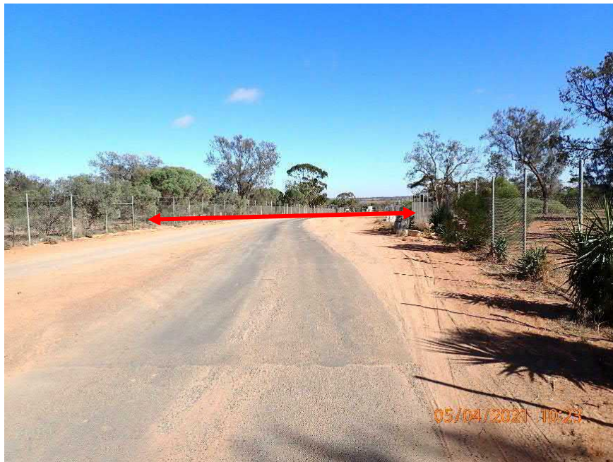
Photograph 02: View of all-weather entry exit road being in excess of 16m in width.
