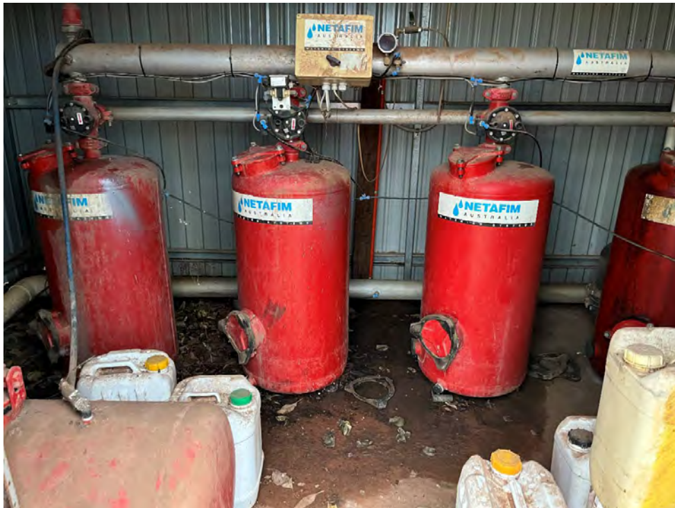
Photo 17. Lot 1 DP1269246 Inside former pump and chemical storage shed
