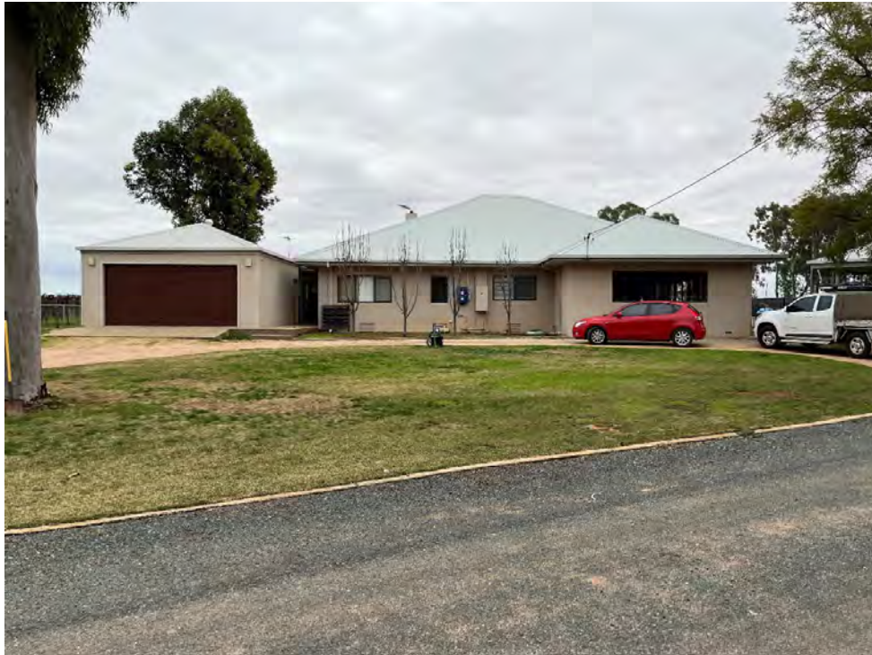
Photo 27. Lot 2 DP1200627 View of residence
