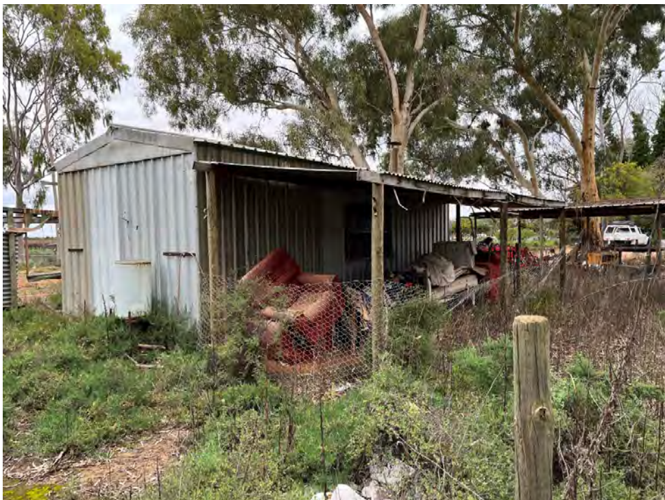
Photo 36.: Lot 3 DP236223 Shed unable to be accessed
