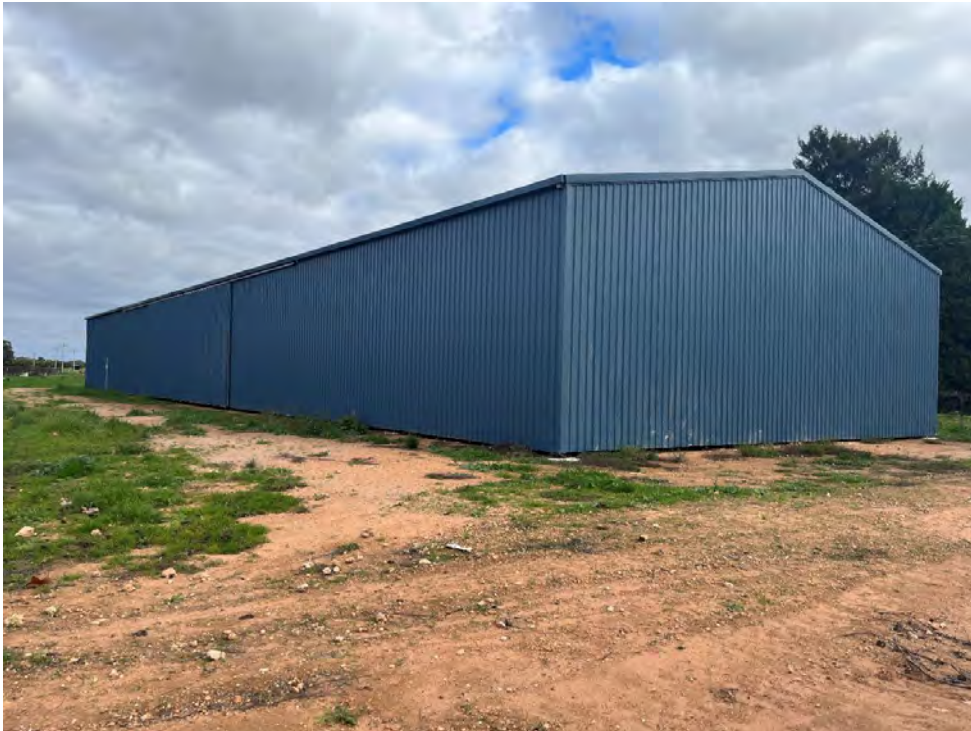
Photo 19. Lot 2 DP1152903 Large vehicle, chemical and general storage shed
