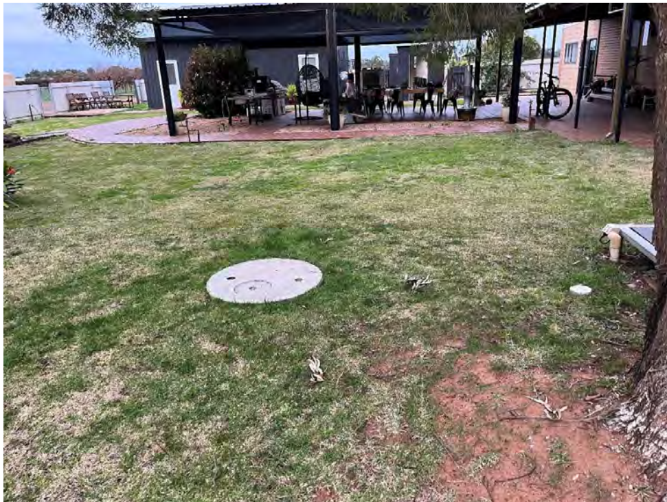
Photo 7. Lot 1 DP1152903 View of one of two septic tanks located at the rear of the land parcel
