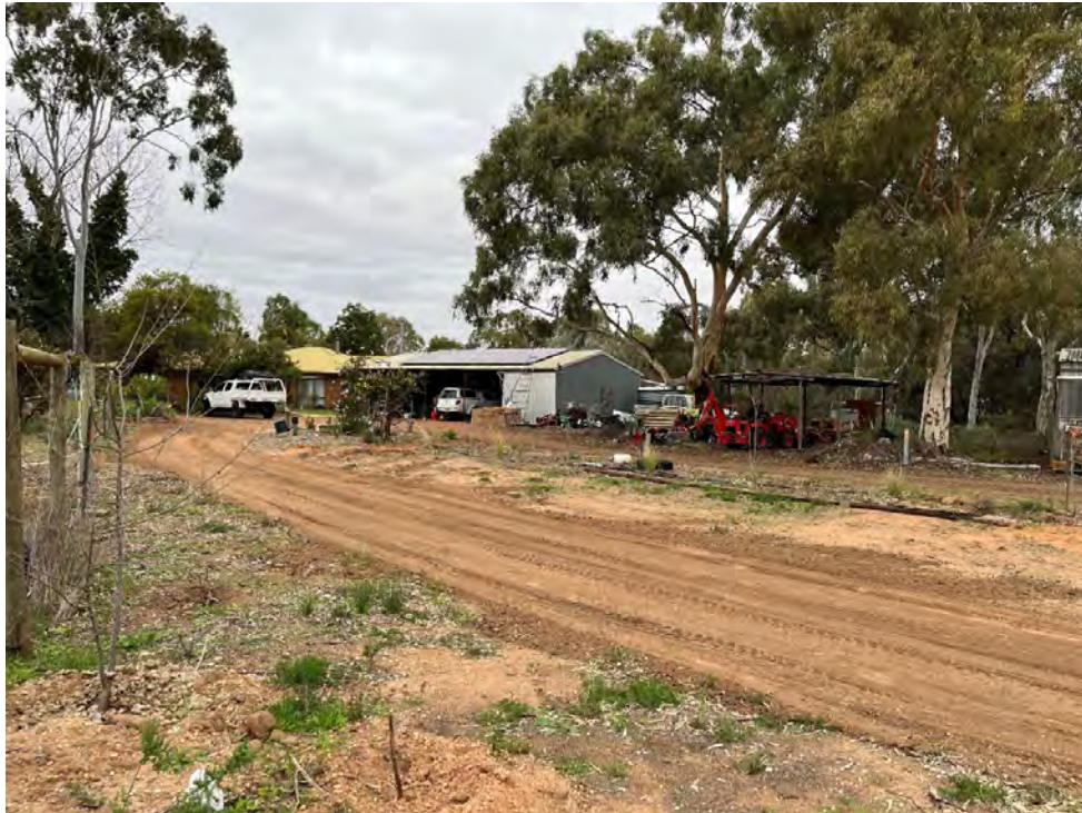
Photo 28. Lot 3 DP236223 View of residential dwelling, shed and carport
