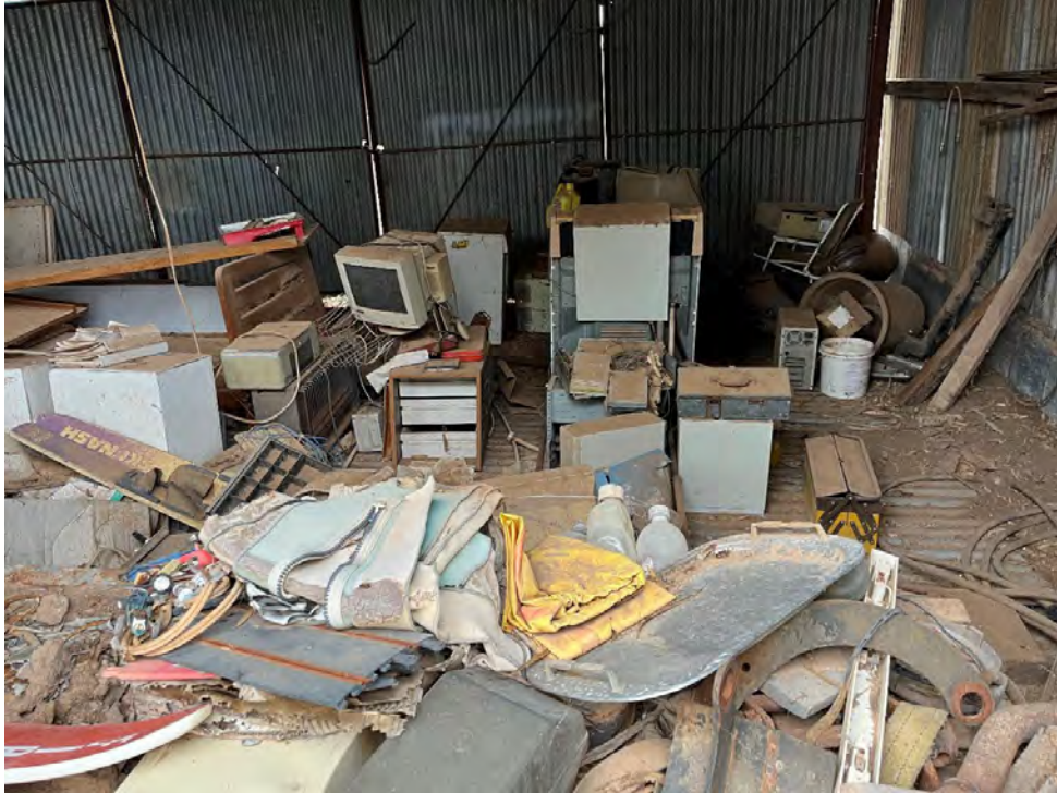
Photo 30. Lot 3 DP236223 View inside dilapidated storage shed
