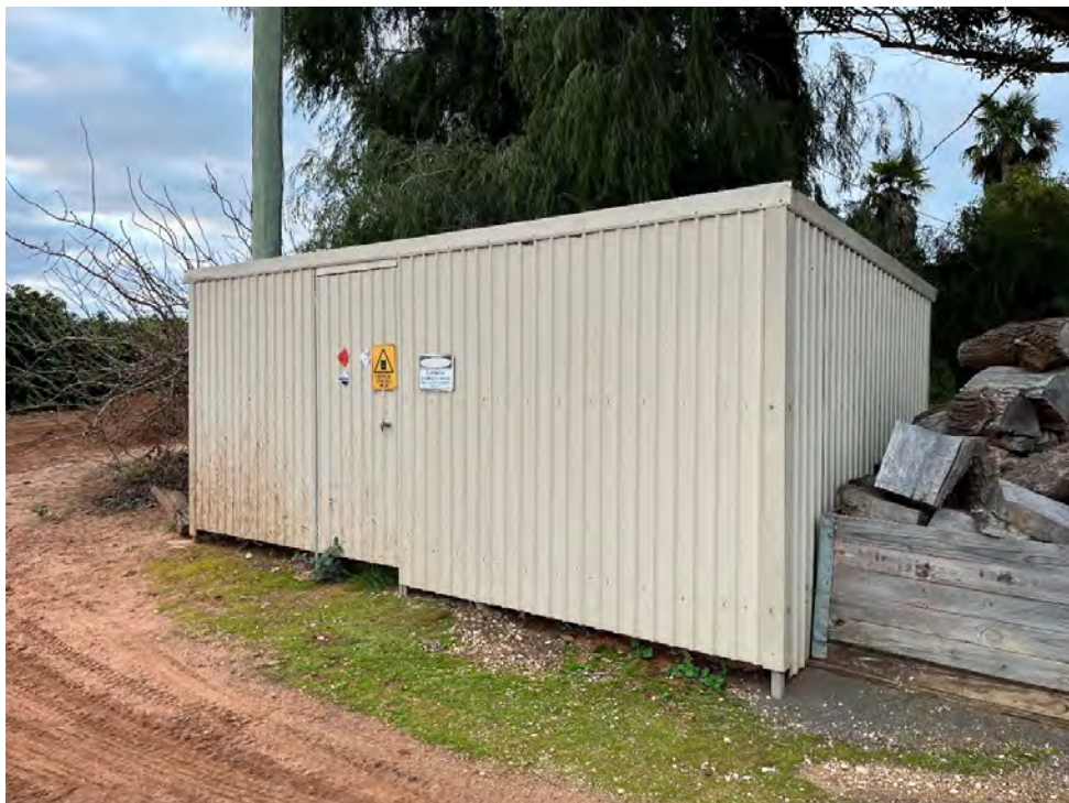
Photo 16. Lot 1 DP1269246 Former pump and chemical storage shed
