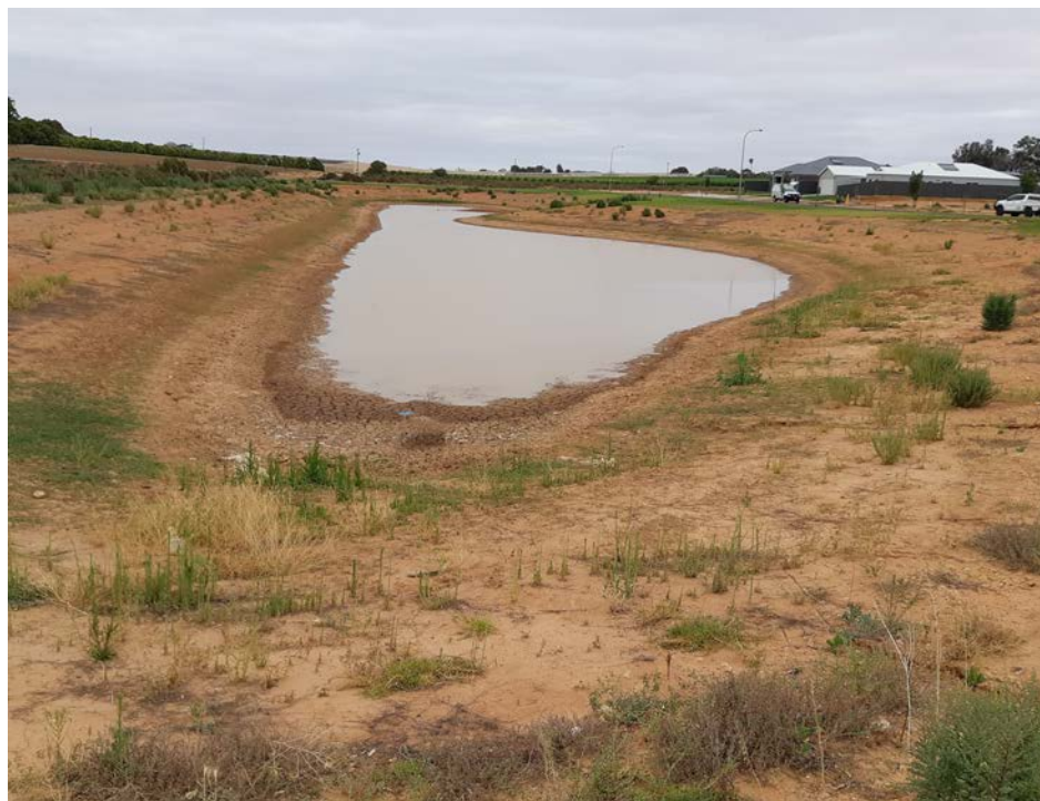
Retention Basin at Livingstone Drive
