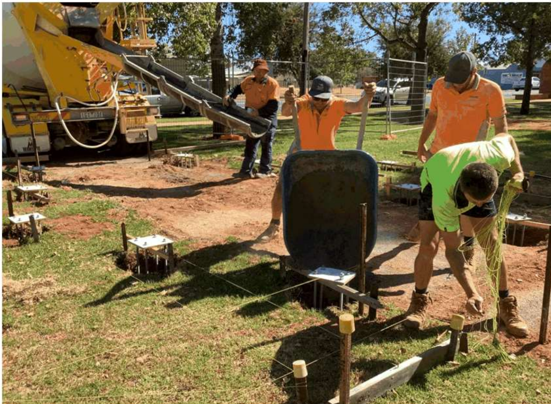
Dareton Travellers Rest – pouring concrete for footings - 5/11/21
