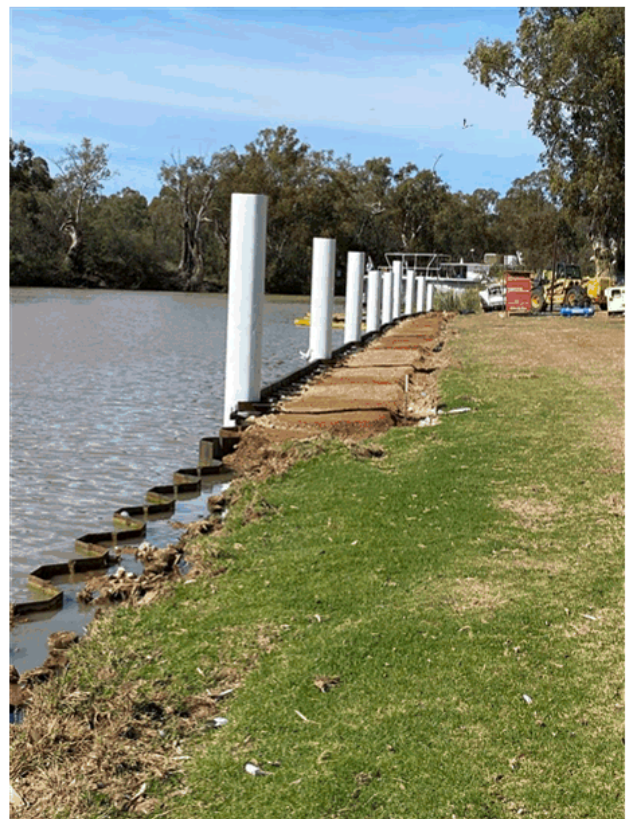
Wentworth Riverfront – installation of sheet piling for houseboat mooring area and houseboat mooring area progress
