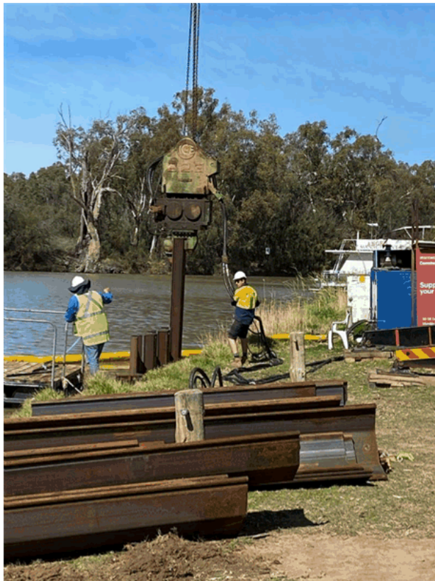
Wentworth Riverfront – installation of sheet piling for houseboat mooring area and houseboat mooring area progress
