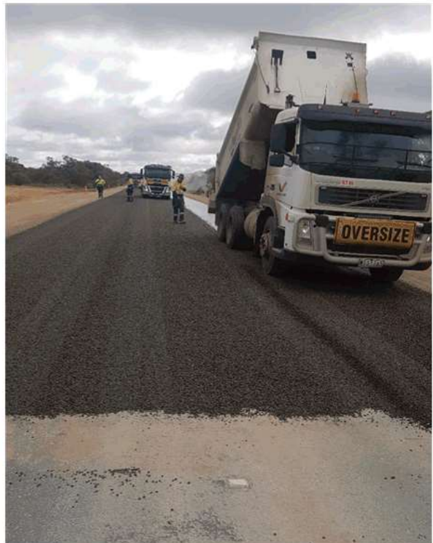
Segment 40 - Sealing work 4/08/2021
