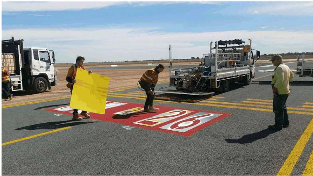
Image 7 – completion of the linemarking works 7/04/21
