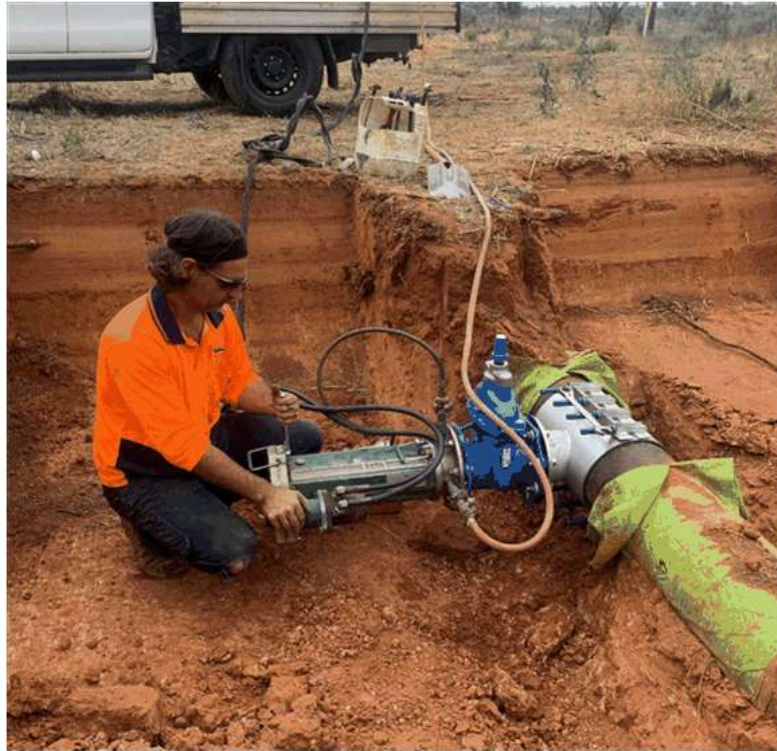
Mourquong Water Main Extension - Live tapping of main 12 February 2021
