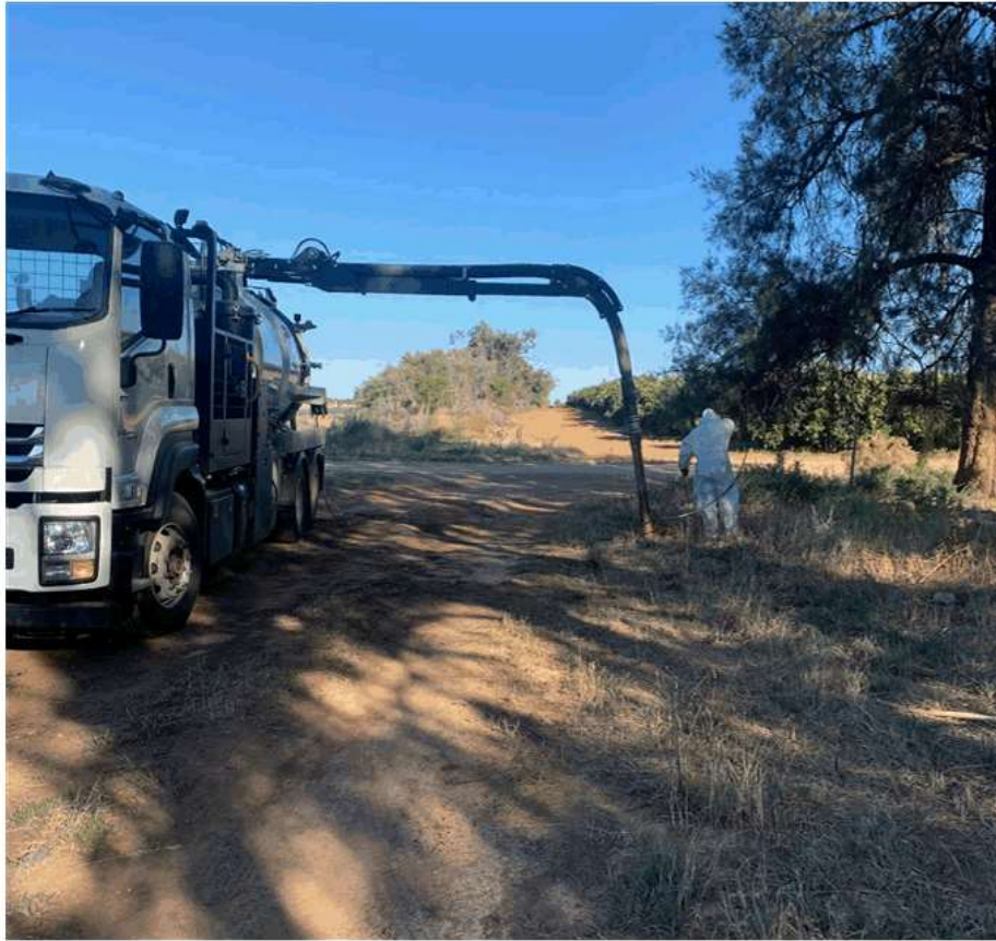
Image 6 – Hydro vac under way at Mourquong Water Main Extension
