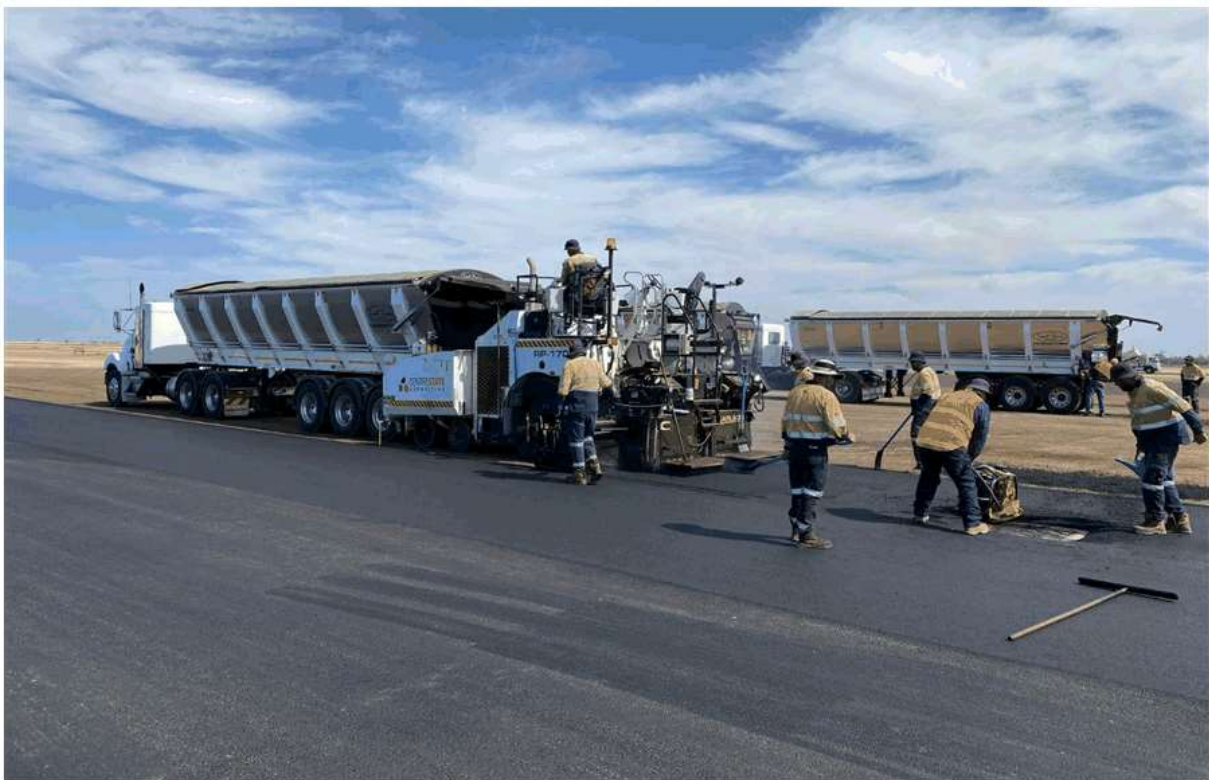
image 32 & 35 - Sealing and asphalt works underway at the Wentworth Aerodrome
