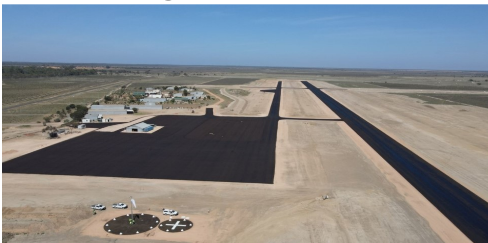
Drone image shows Wentworth Aerodrome upgrade progress
