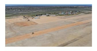
Construction of the runway, taxiway and apron area was completed in August, with installation of the lighting and electrical upgrades to commence in September. Photo shows material stockpile site, pug mill and grader working alongt he runway strip
