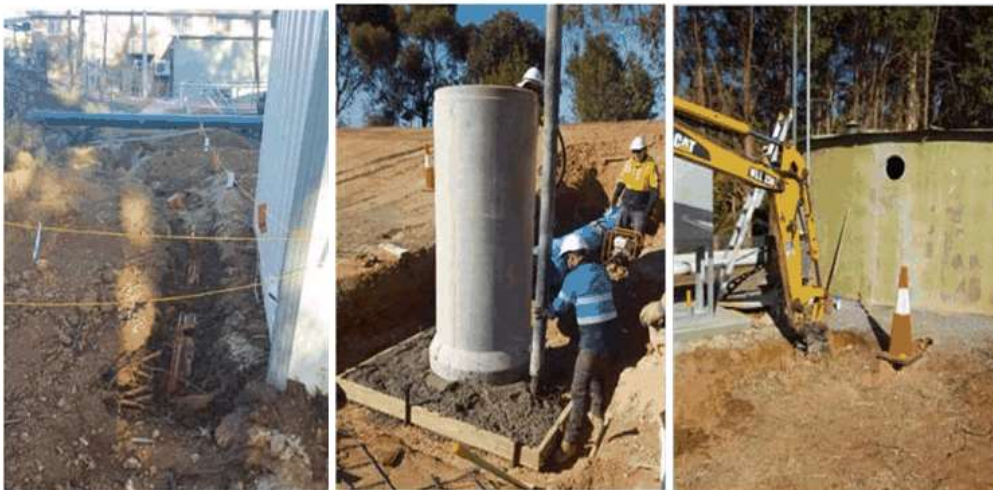
Image 13 – Gol Gol WTP replacement of inlet structure on Lagoon 2 and footings work at the balance tank
