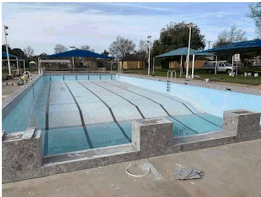
Image 2 – Dareton lap pool tiling works in progress
