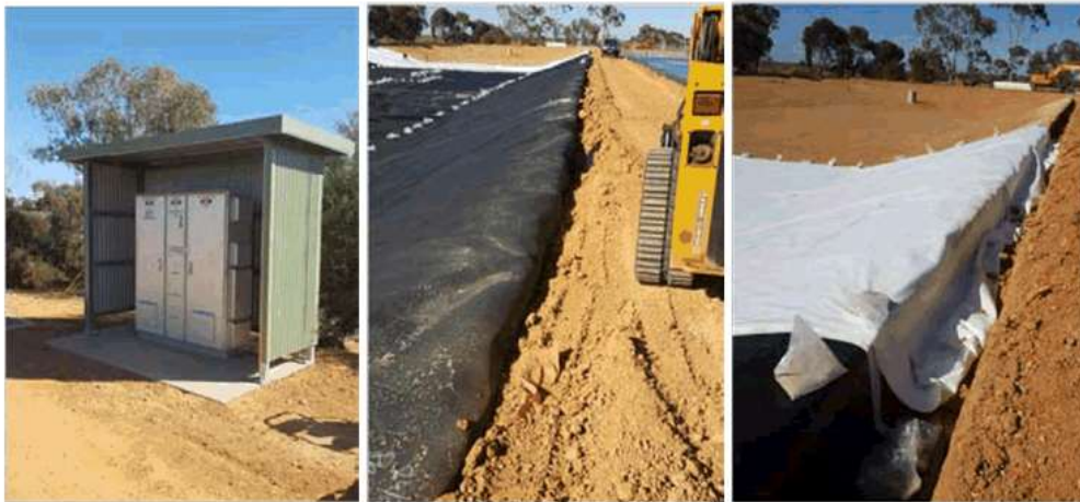
Image 14 - Gol Gol WTP switchboard and installation of HDPE liner at pond 2
