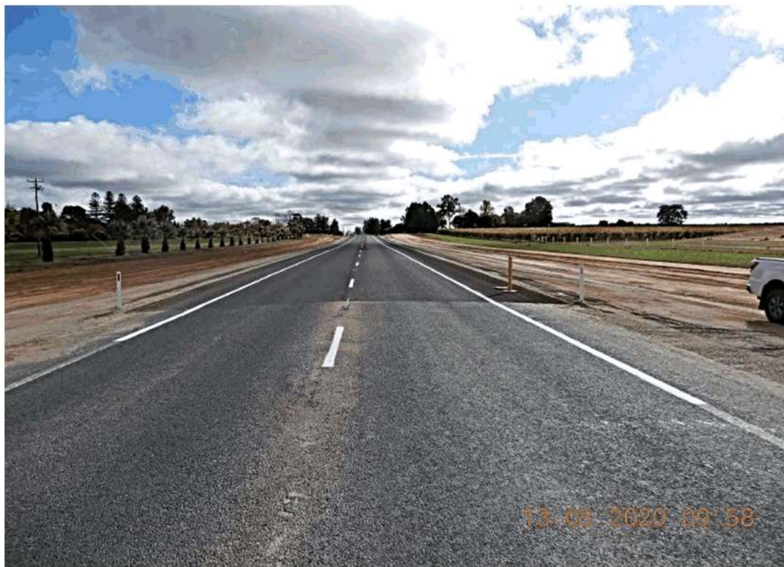
Image 8 – Segment 130 Sturt Highway Trentham Rehabilitation new Linemarking
