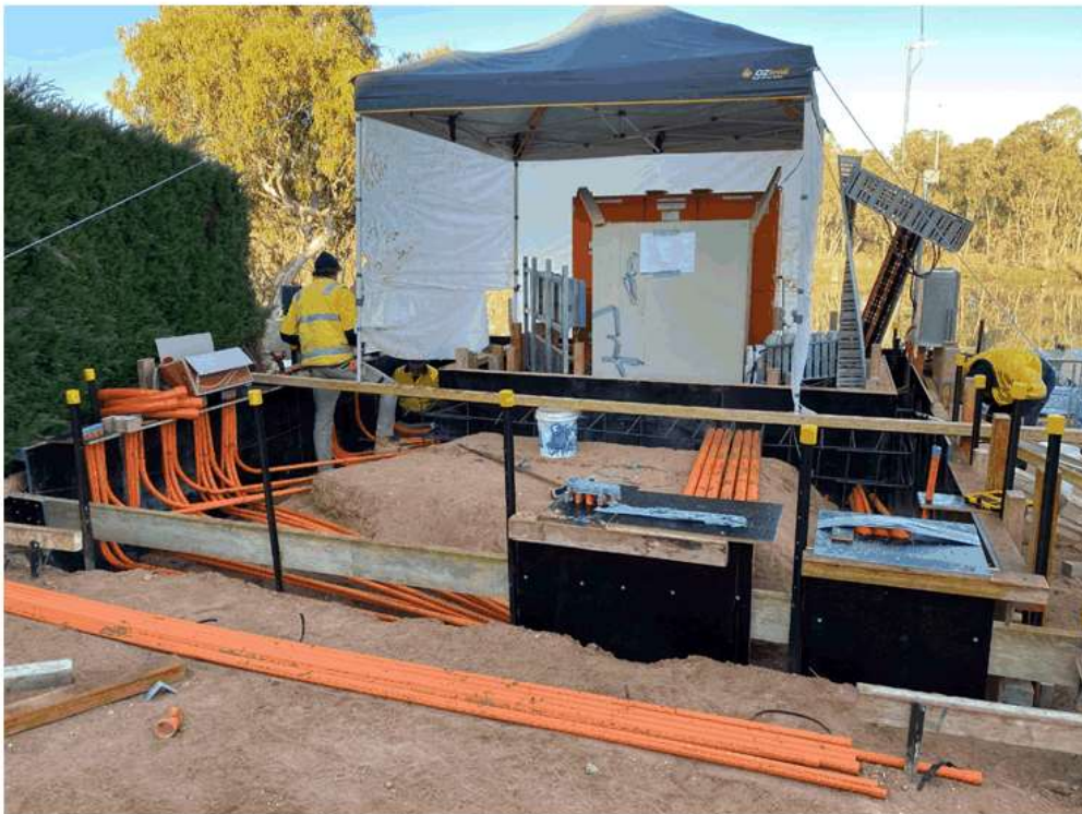
Image 2 - Gol Gol Water Treatment Plant construction of raw water pump station
