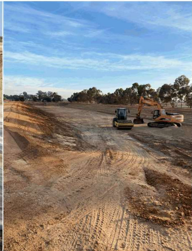
Image 6 - Gol Gol WTP Lagoon 2 liner construction
