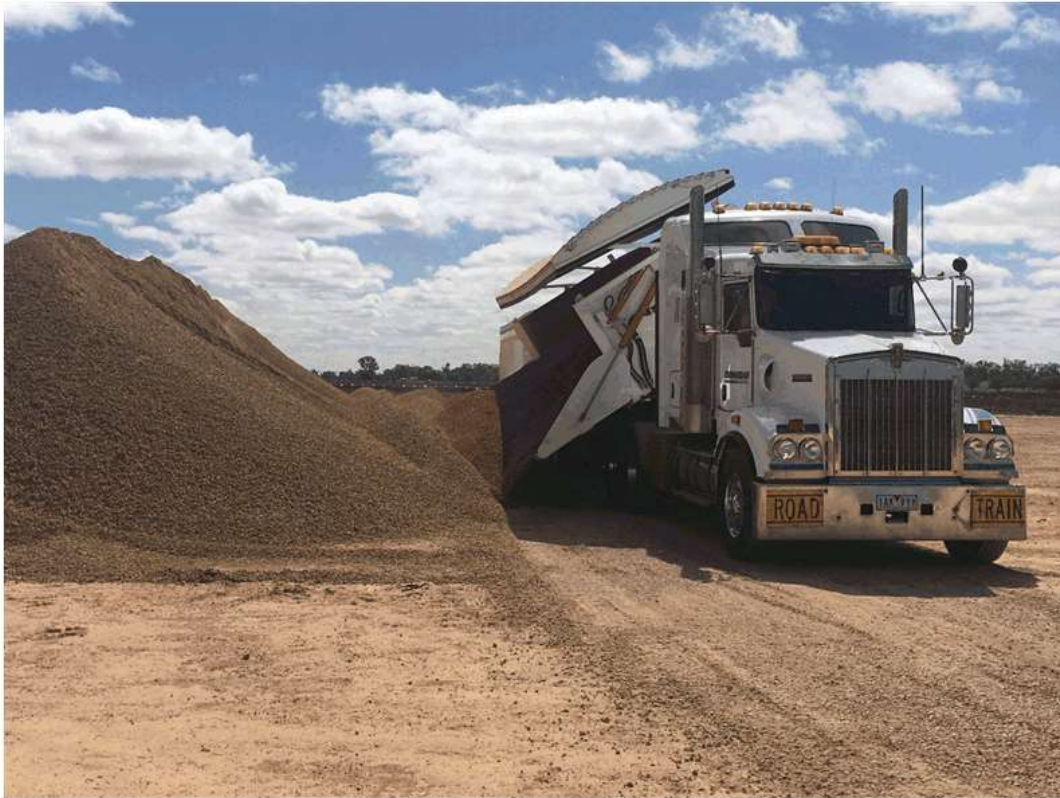
Image 7 – Wentworth Aerodrome stockpile site delivery of Class 3 material for runway construction
