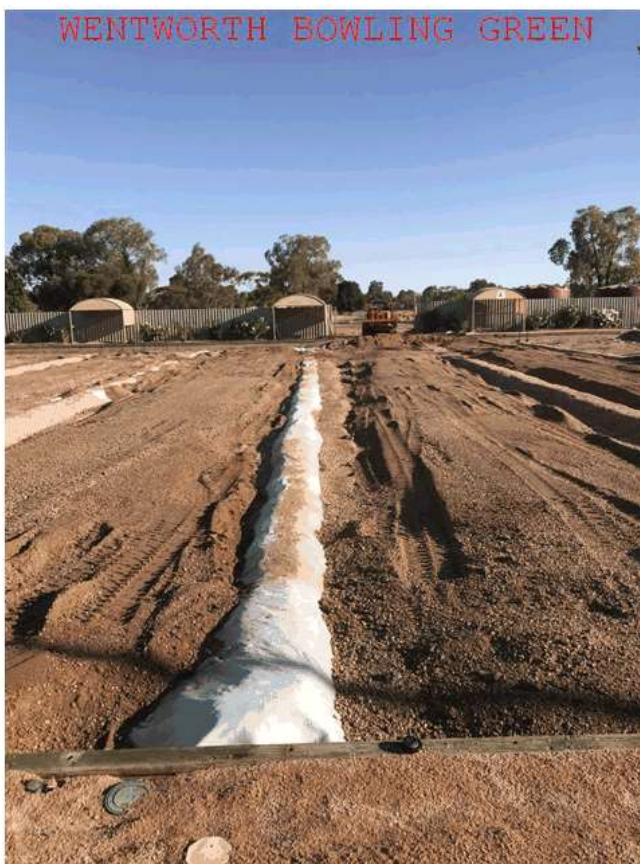
Image 14 – Installation of the Geo-Fab
