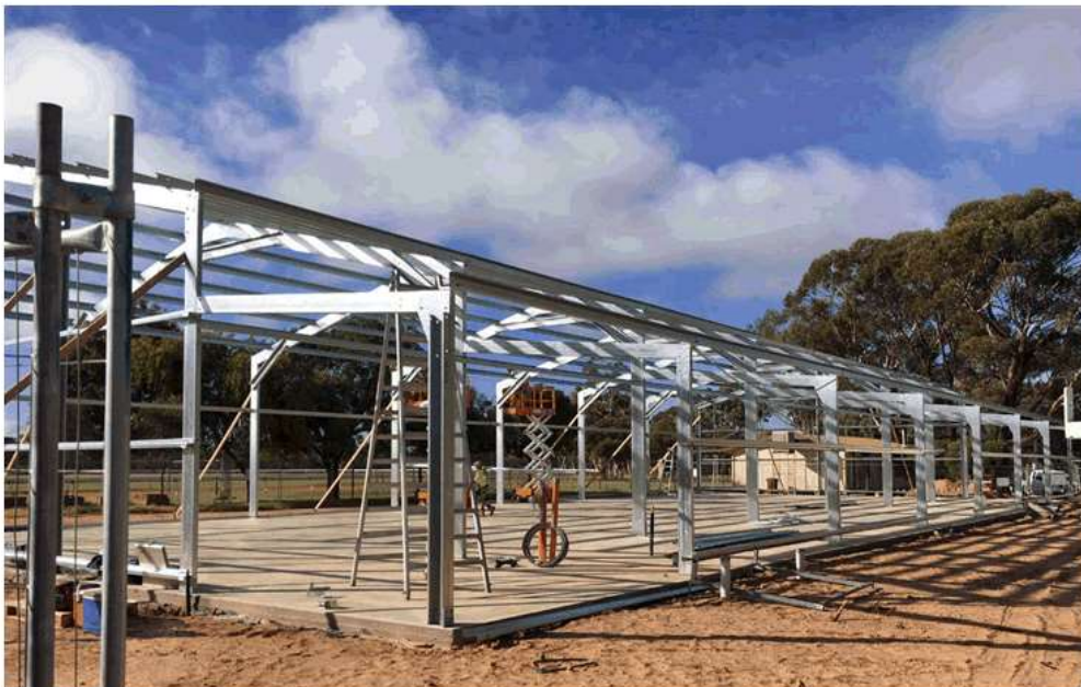
Image 6 – Barrett Pavilion erection of the steel frame
