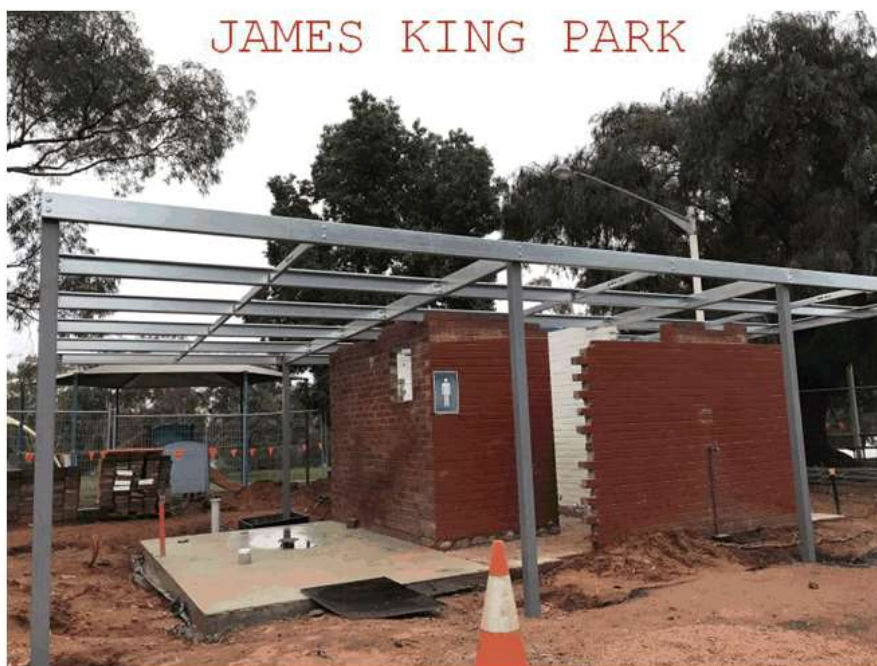
Image 15 – James King Park construction of new roofing
