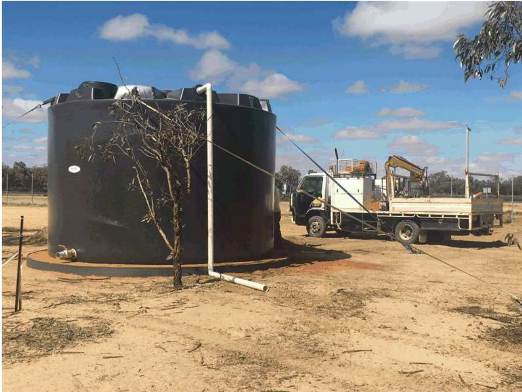
Image 9 – Wentworth Aerodrome installation of new 50,000 litre poly tank
