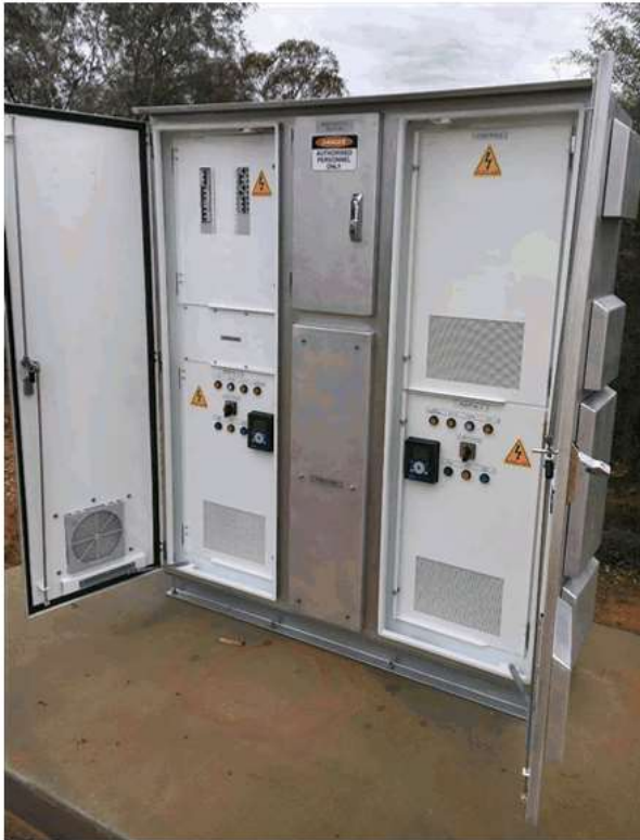
Image 14 – Gol Gol Water Treatment Plant – VSD and switchboard installation
