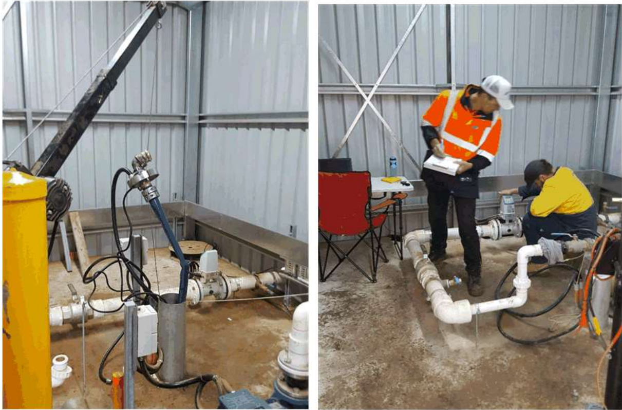
Image 10 & 11 – Pooncarie Bore Upgrade Pump Testing
