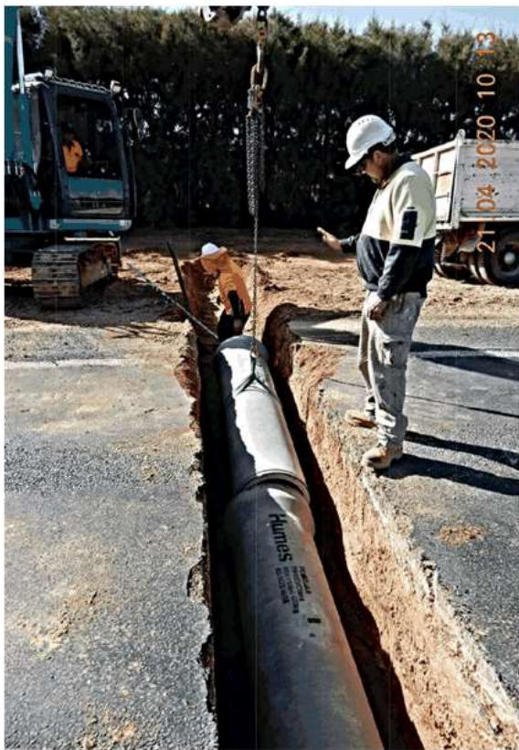
Image 3 & 4 – Sturt Highway Reconstruction - Segment 130 - Earthworks and installation of drainage pipe
