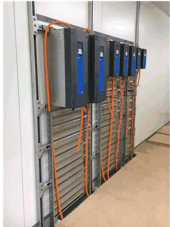
Image 14 – Gol Gol Water Treatment Plant – VSD and switchboard installation
