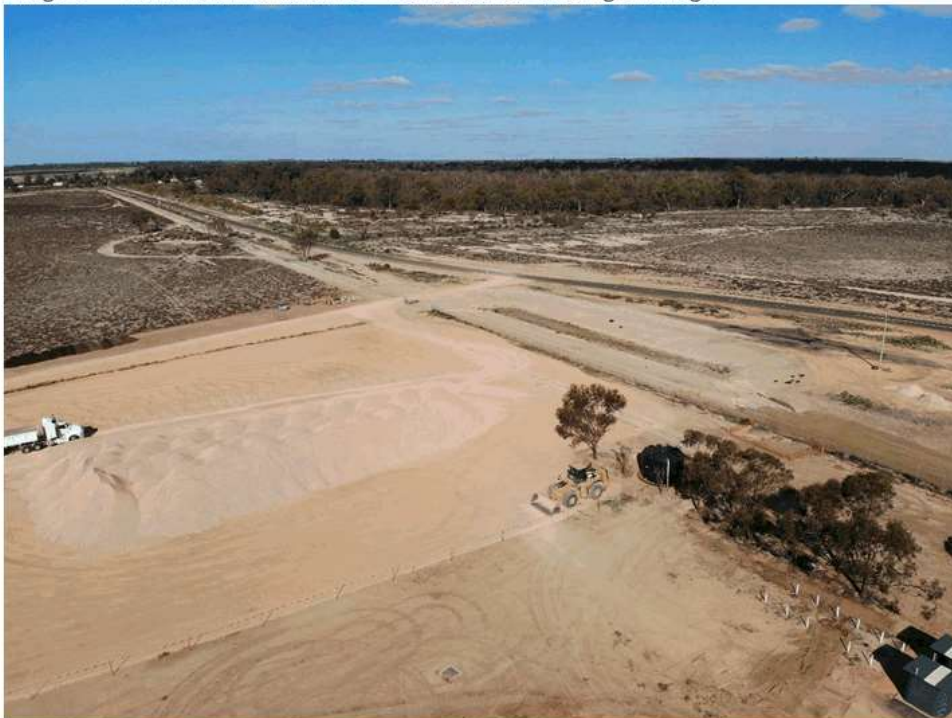
Image 6 – Wentworth Aerodrome – Stockpile Site Class 3 material for runway
