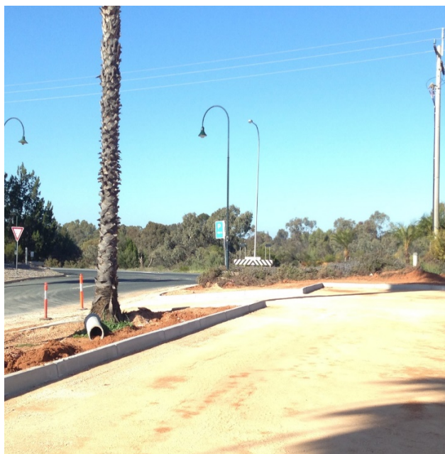
Main carpark kerbing completed and base course of road pavement ready for sealing. Drainage in place and connected to drainage outfall.
