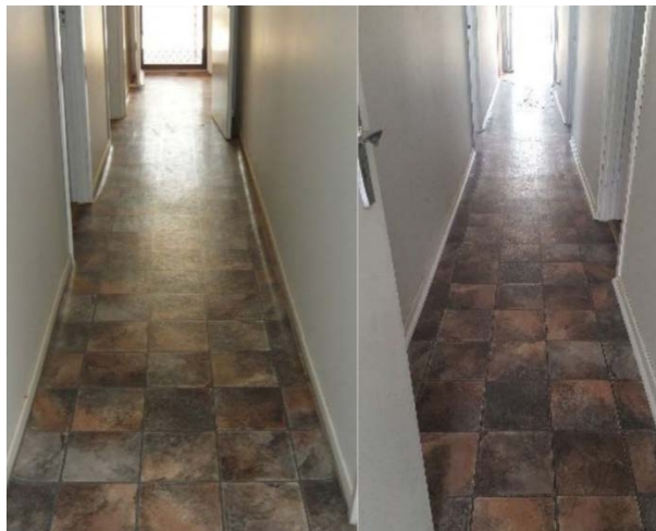
Lino peeling throughout the building has been re-attached to the floor with use of quads
