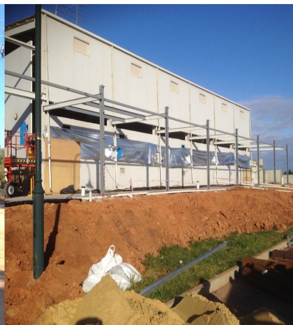
Steelwork under erection to western side. Note existing wall still in place to render weather protection and security (since removed as outer wall installed).
