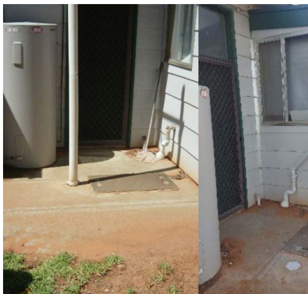
Outdoor waste pit was capped off and external pipe was attached to kitchen drainage
