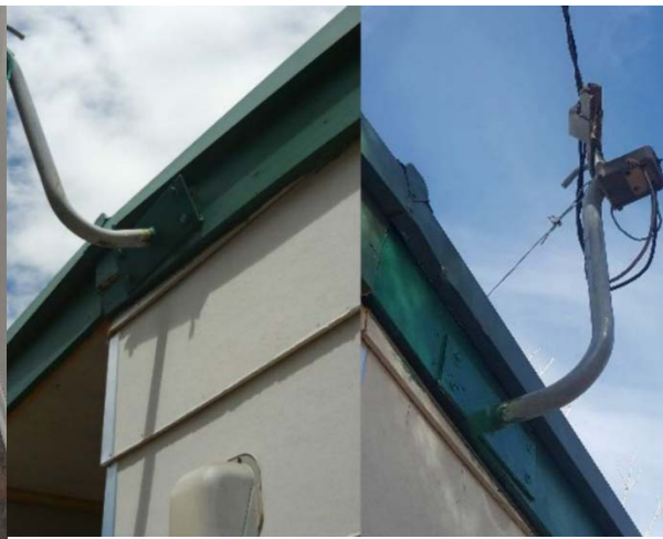
Powerline connected to fascia was deteriorating, and has been repaired
