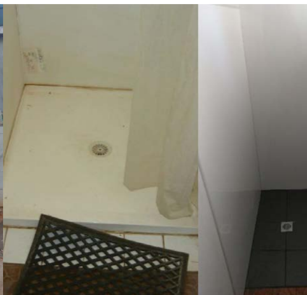
Shower draining issues with water leaking out the side of the building and front of the shower basin was rectified
