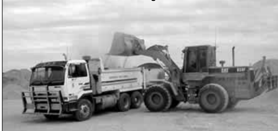
A Shire maintenance crew loads gravel for road maintenance
